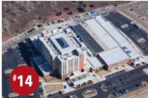
➤ Saratoga Roofing & Construction of Oklahoma City roofed the Embassy Suites and Convention Center in Norman, Okla. Photo courtesy of Saratoga Roofing & Construction.
