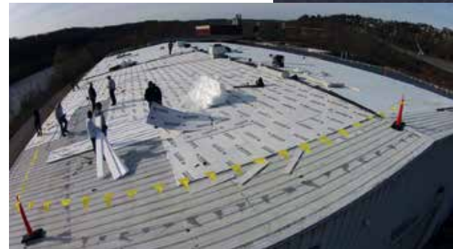
Luck works on a project at P&I Partners, Donora, Pa.
